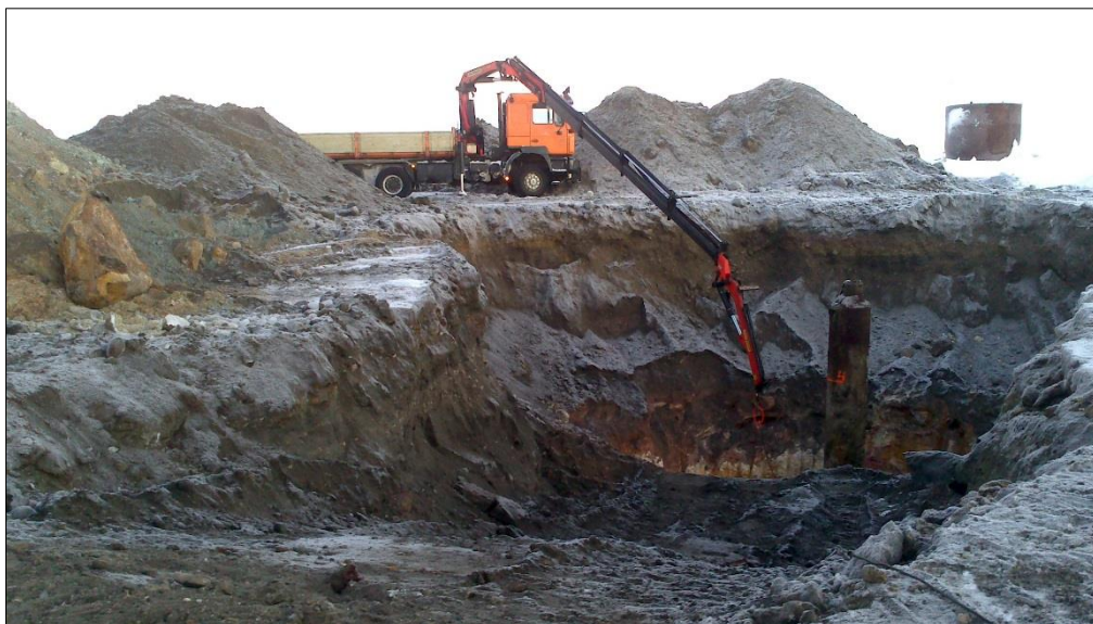
Figure 2.2.3. Picture showing the retrieve of the uppermost 8 meters of the IDDP-1 wellhead for inspection (Photo from the National Power Company – Landsvirkjun).
