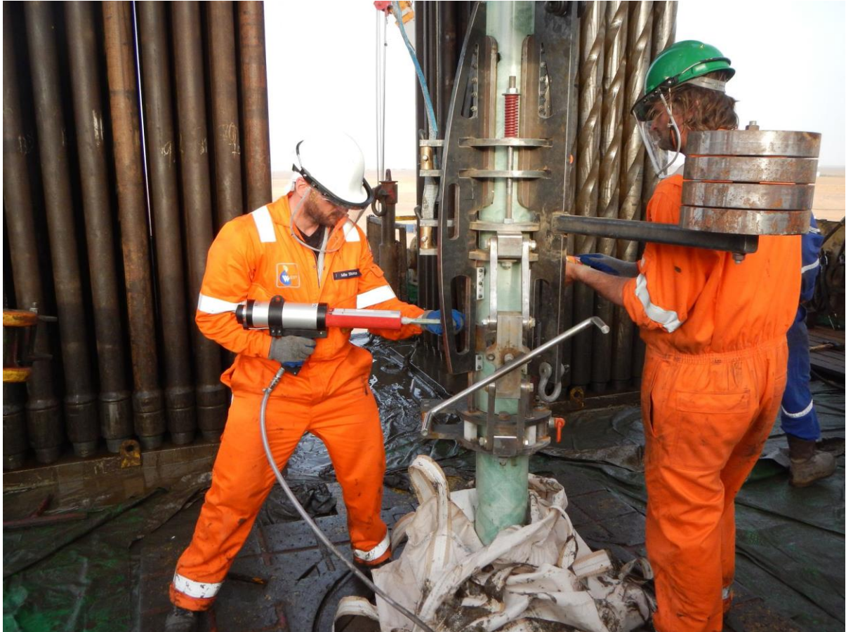
Figure 6: Making the on-site adhesive connection
