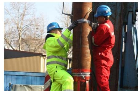
Installation of a fibre optic cable behind casing in a low temperature well in Berlin.
